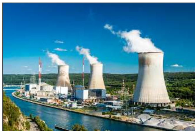
Cooling water control for power plants
